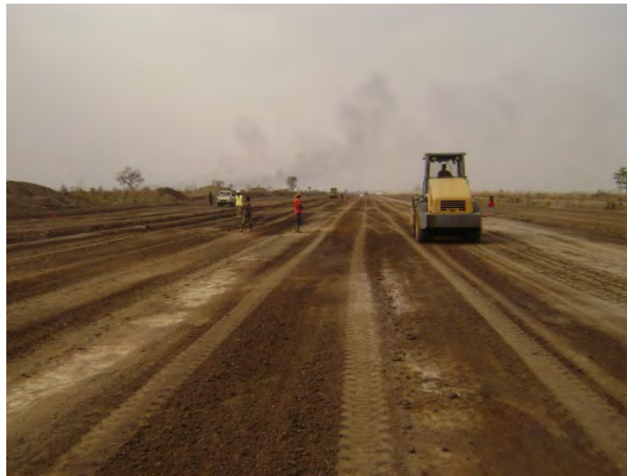
Figure 7: Canal compaction using vibrating sheep foot roller machine
