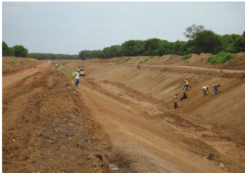
Figure 8: Canal bed preparation and trimming
