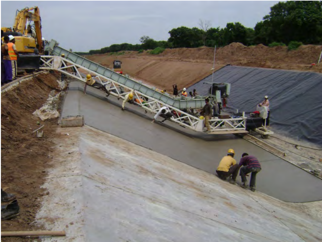
Figure 12: Finishing process for concrete Lining
