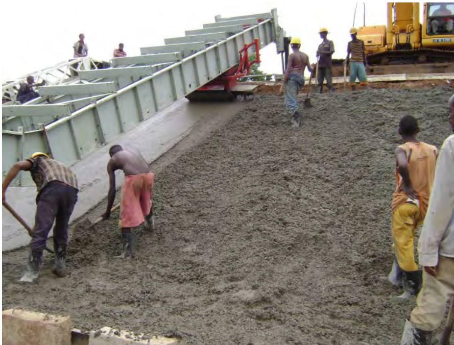
Figure 11: Casting concrete on canal side slope
