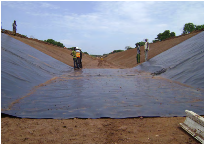
Figure 9: Geo-membrane installation in main canal
